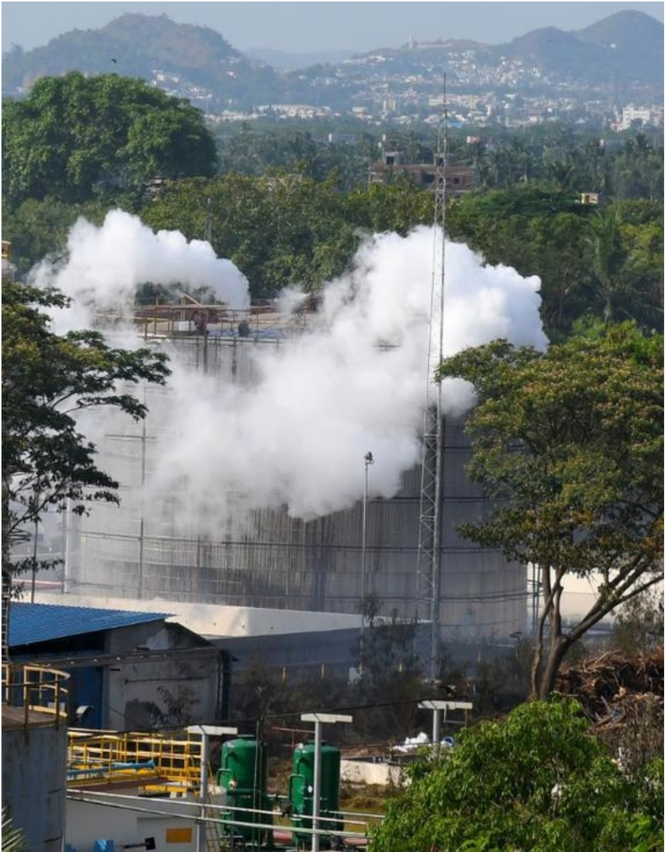
Gas leak in LG Polymer Plant, Visakhapatnam . 07 May 2020 (Source: The Hindu)
